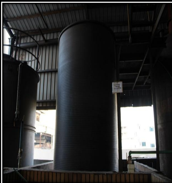
Machinery Name: Settling Tank Location In Plant: ETP Capacity: 50000LTR Use: In Etp for Effluent Storage After Treatment
